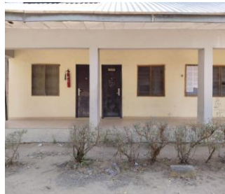
Figure 9: A block of 8 Professorial Offices with a canteen built by the Faculty during my tenure
