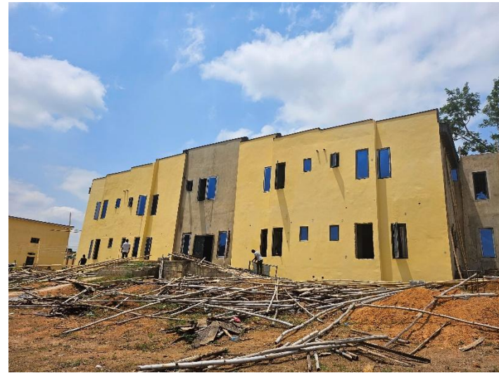
CONSTRUCTION OF HOSTEL AT NIGERIA INSTITUTE FOR SECURITY STUDIES (LOT 1)
