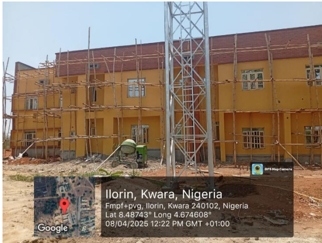
CONSTRUCTION & FURNISHING OF FACULTY OF SOCIAL SCIENCES BUILDING
