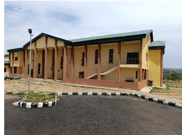
FACULTY OF ENGINEERING 500-SEATER CAPACITY LECTURE THEATRE
