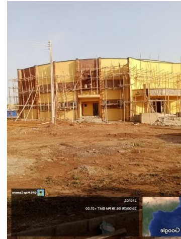
CONSTRUCTION & FURNISHING OF ENGLISH DRAMA STUDIO
