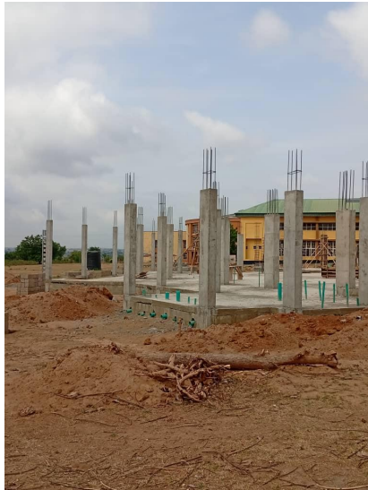
CONSTRUCTION AND FURNISHING OF LECTURE THEATRE (COHS)
