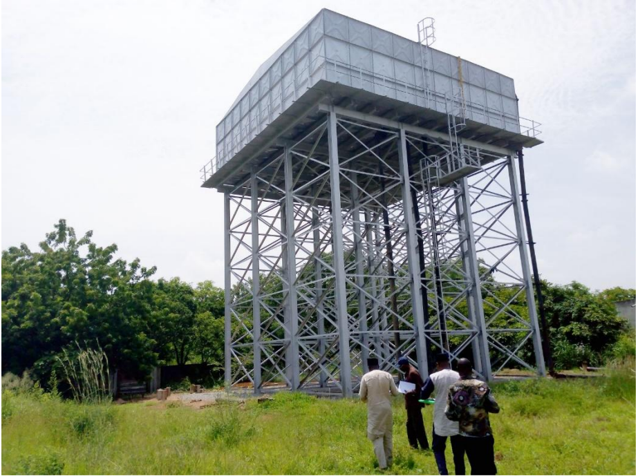
500M Cubic Elevated Pressed Steel Braithwaite Type Water Tank
